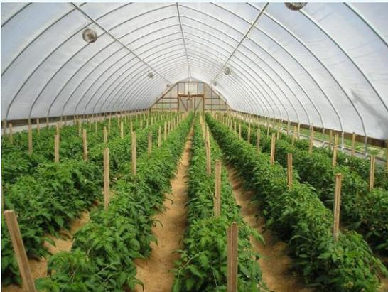
**Hoop house** - a structure made by bending metal hoops or pipes in a semi-circle shape to provide the roof, covered with plastic.
