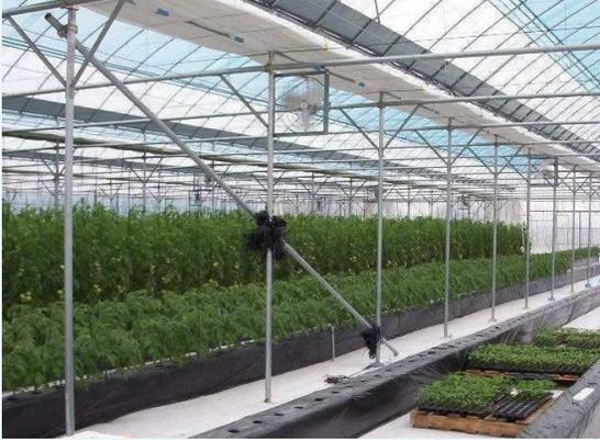
**High tunnel** - a structure covered with clear plastic; originally referred to a structure without auxiliary heat or ventilation, now high tunnels may have this mechanization.
